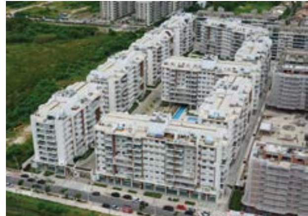
FRAMES RESIDENCE RECREIO DOS BANDEIRANTES
